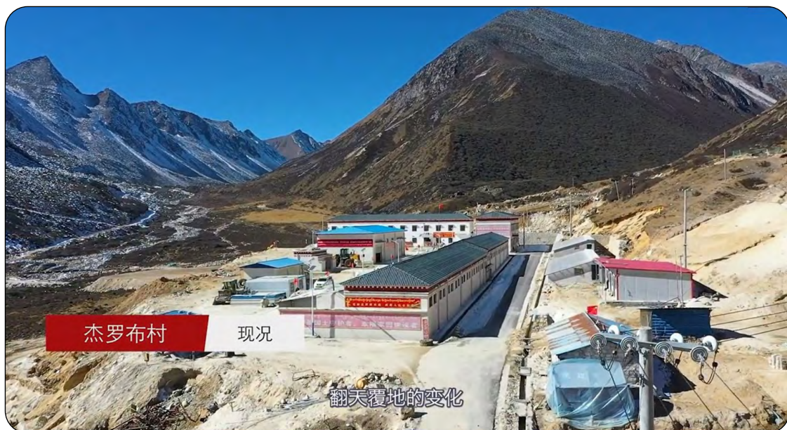
[Fig. 19. The village of Jieliubu after Phase 1 construction was completed in October 2018. Four additional blocks with 20 more homes were added in Phase 2. Screenshot from a video that aired in December 2020. Credit: TAR Internet Information Office. URL: http://news.xhby.net/tuijian/202101/t20210120_6954173.shtml ]
